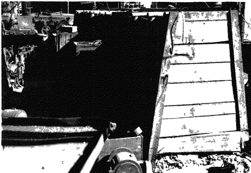
Figure 12.37c. Earth-filled, wooden blast walls protecting machinery (0.85 mile from ground zero at Nagasaki).
